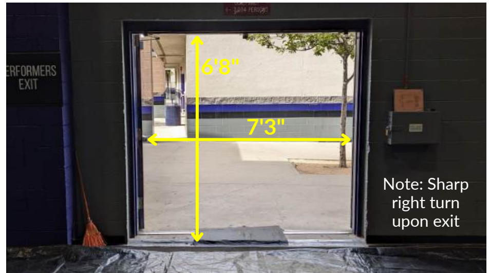
Exit Door (1 double door)
