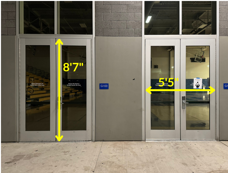
Entry Doors (2 double doors)
