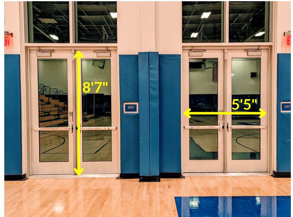
Exit Doors (2 double doors)
