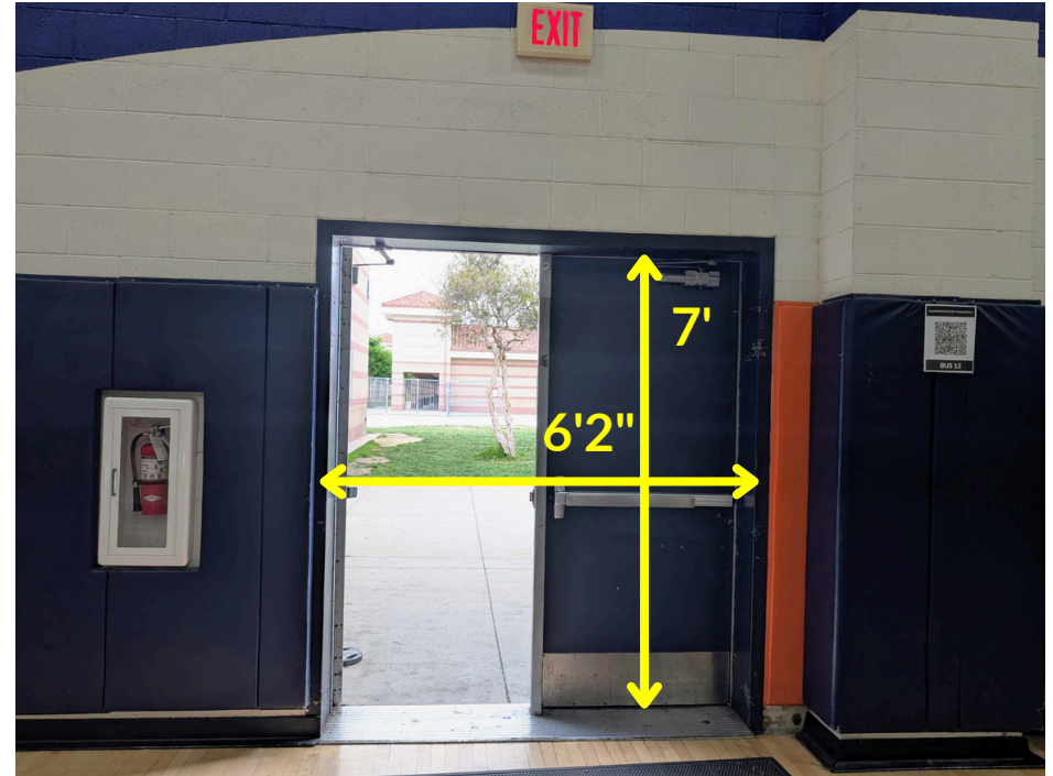
Exit Door (1 double door)
