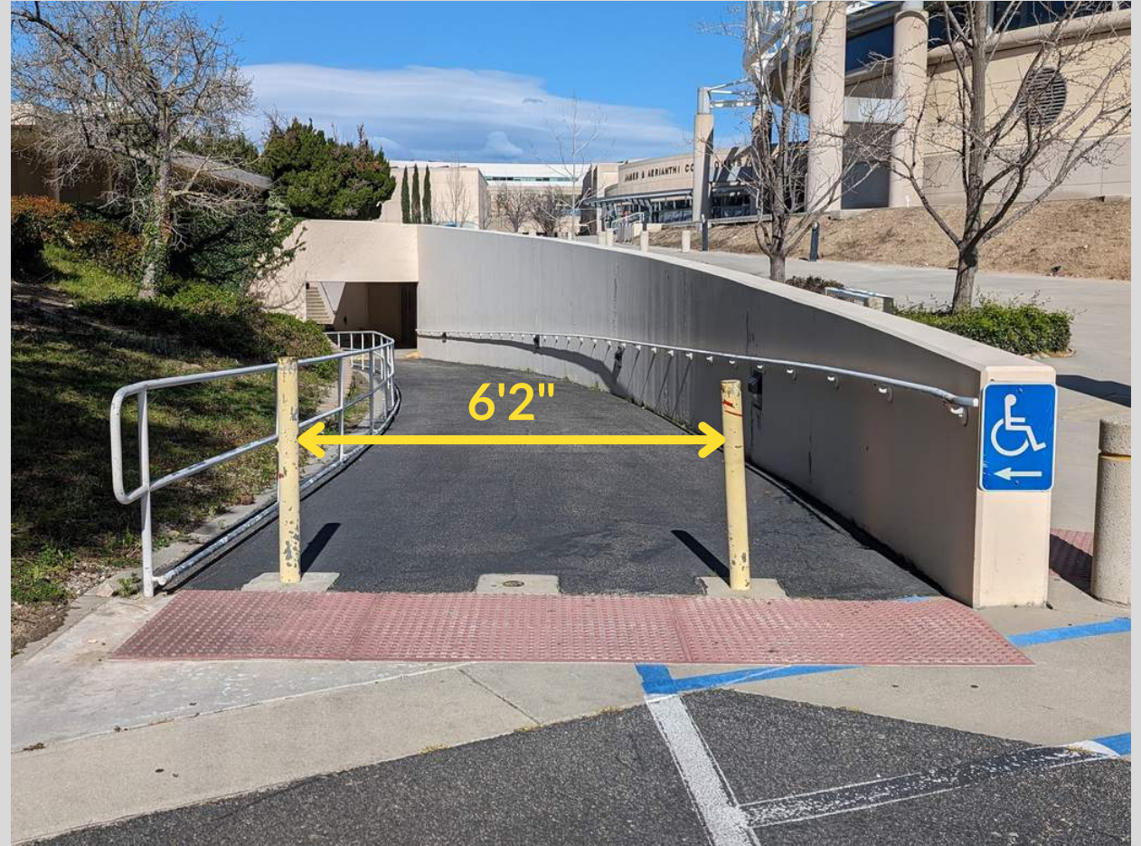
Ramp to Performance Entry
