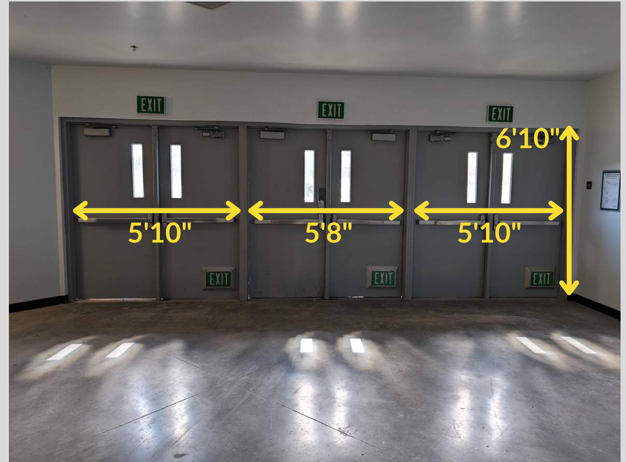
Exit Doors to Floor Folding (3 double doors)
