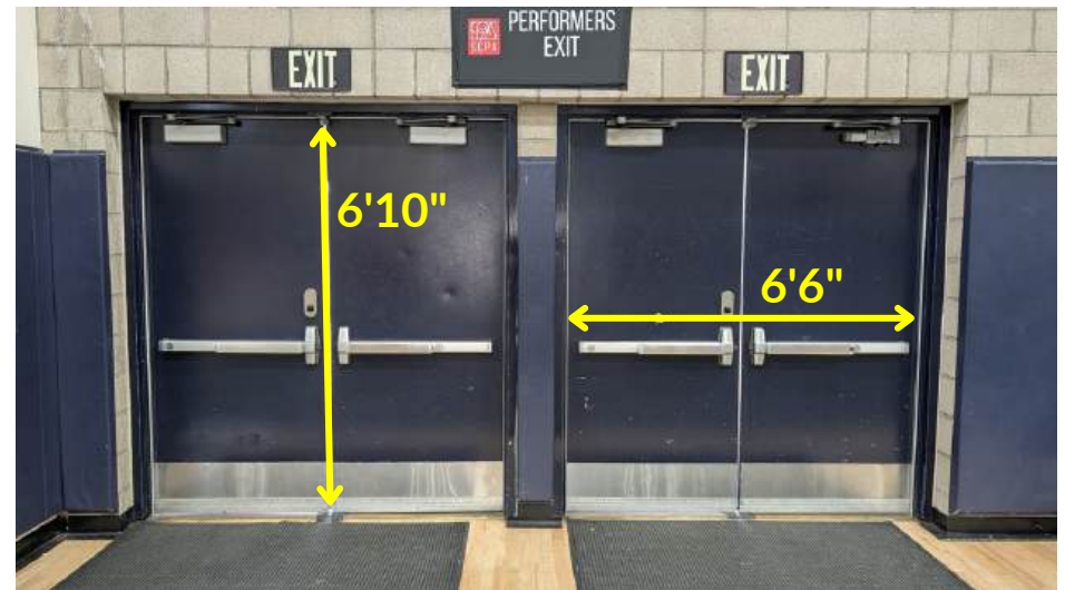
Exit Doors (2 double doors)
