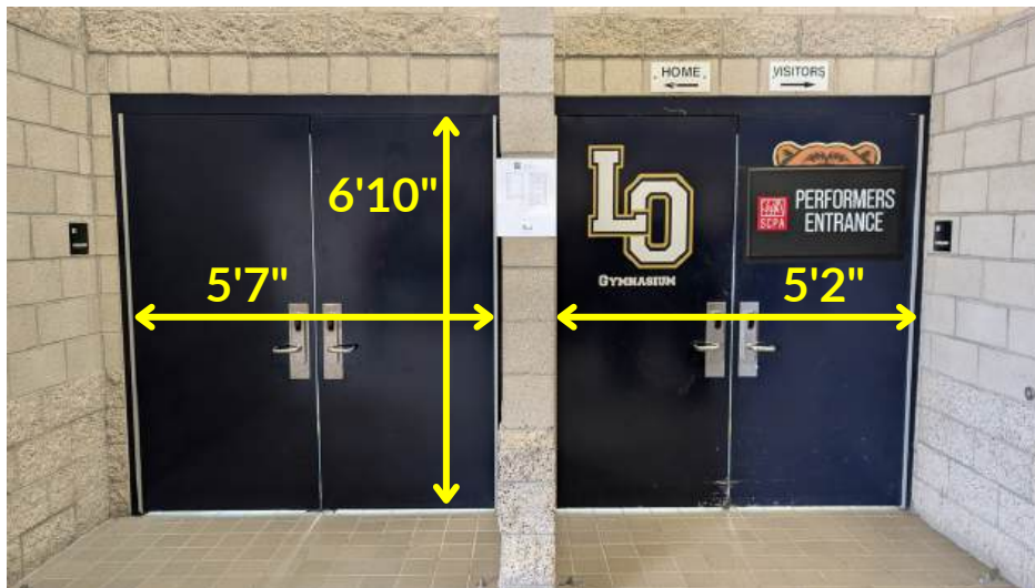
Entry Doors (2 double doors)
