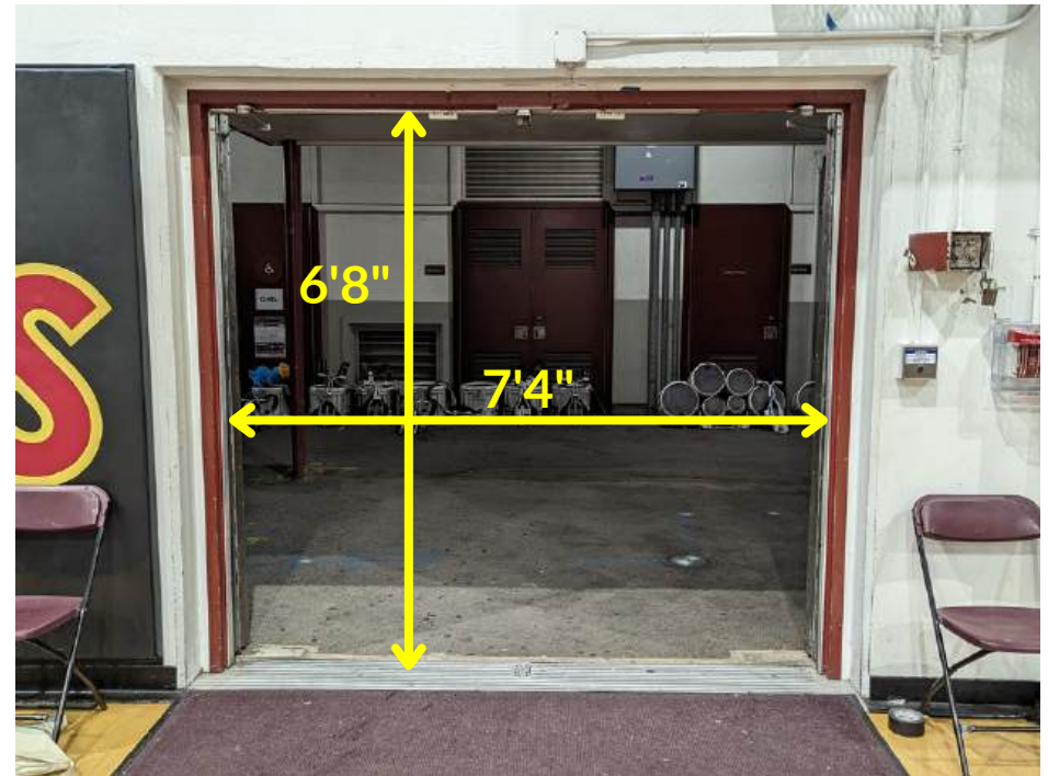
Exit Door (1 double door)
