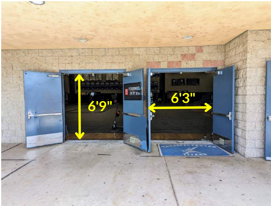
Entry Doors (2 double doors)
