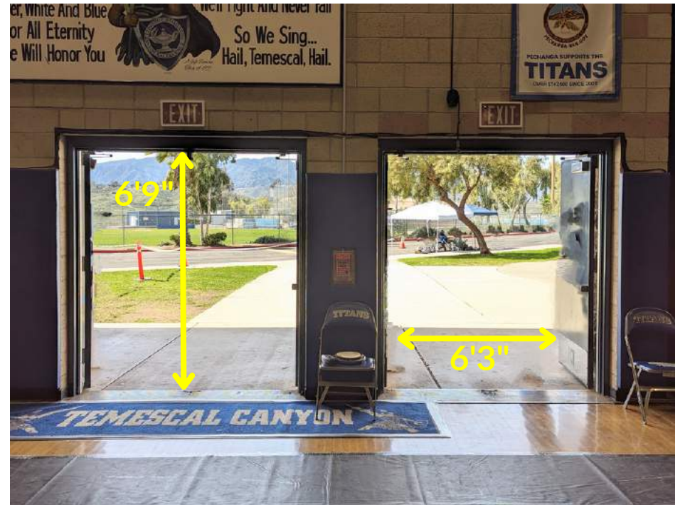
Exit Doors (2 double doors)
