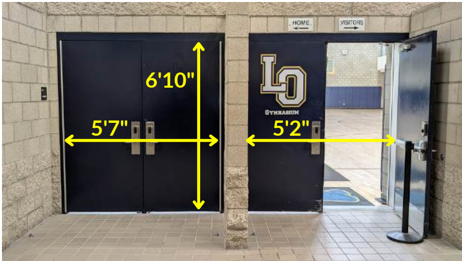
Entry Doors (2 double doors)
