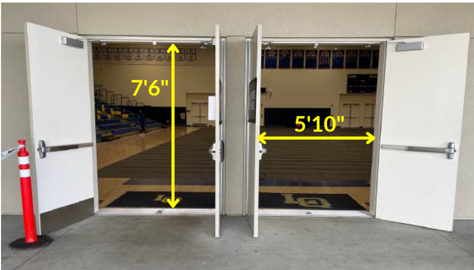
Entry Doors (2 double doors)
