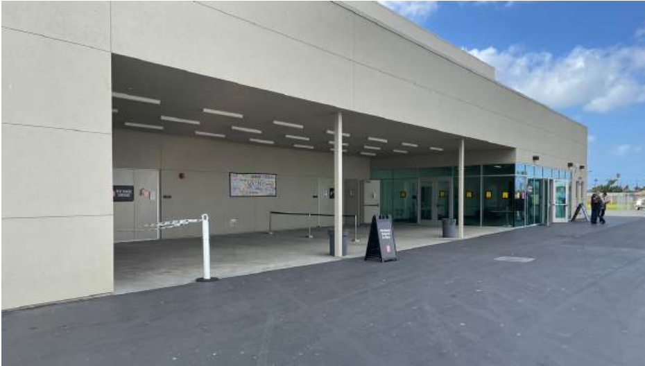
Covered Prestage Area
