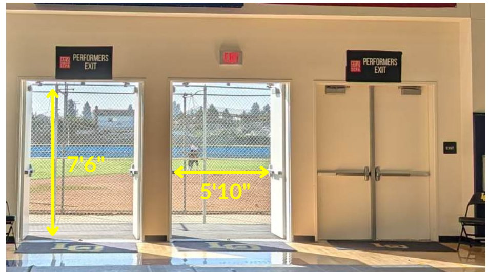
Exit Doors (2 double doors)
