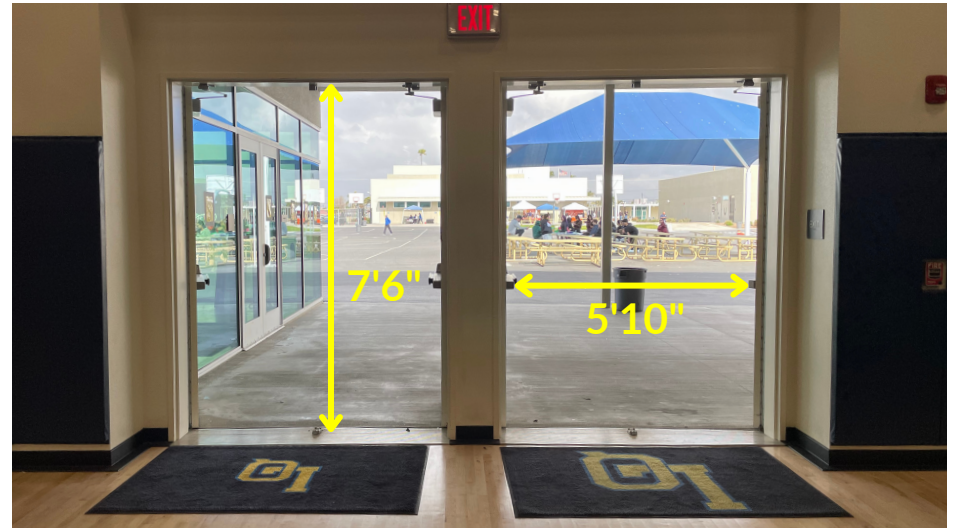
Exit Doors (2 double doors)
