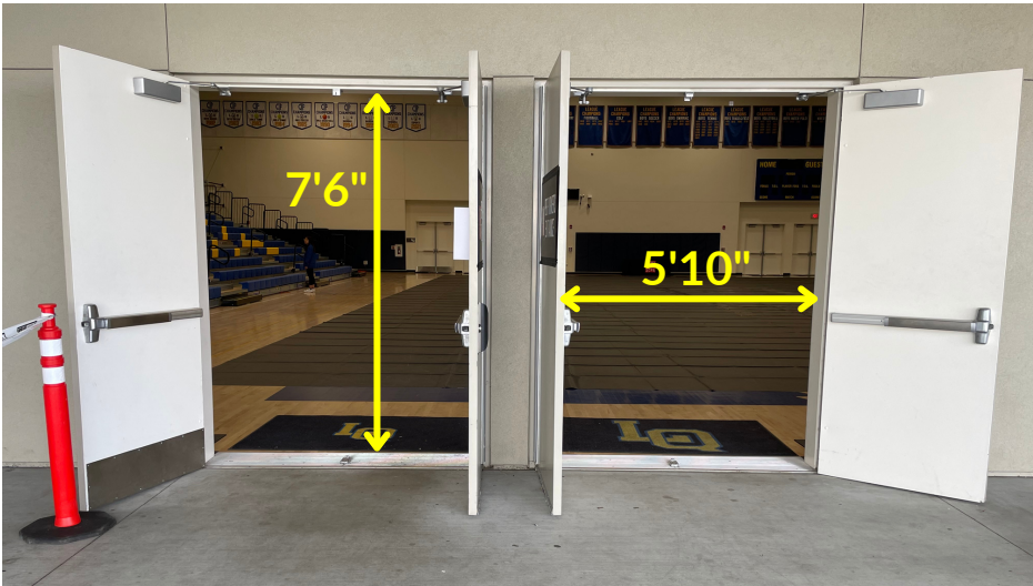
Entry Doors (2 double doors)
