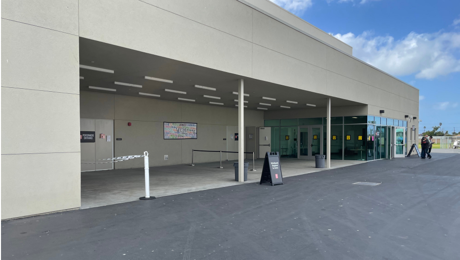
Covered Prestage Area
