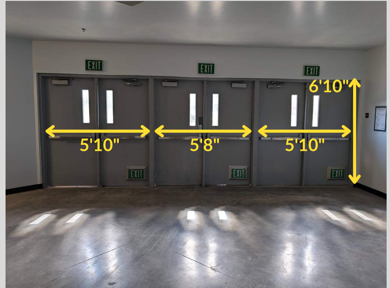
Exit Doors to Floor Folding (3 double doors)
